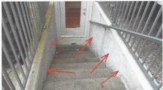
2. Grading: Negative at the front of the house - Maintain a 6-10% slope away from the house for 10 Feet. Always Promote positive (+) drainage away from the foundation and extend run off from roofing and downspouts a minimum of ten feet from the foundation. If this can't be accomplished consider a swale cut or drainage system.
